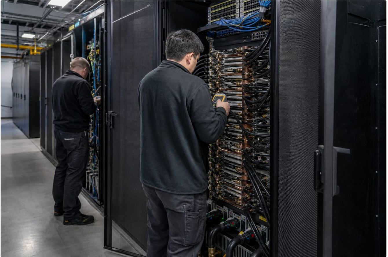
Generated documentary image for TechDirectory Research. The scene depicts a technically plausible direct-to-chip liquid-cooling and scale-out networking installation; it is not a photograph of a named facility.
